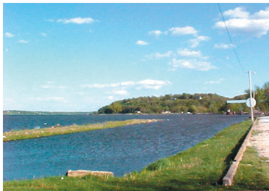
Existing view of Riverfront Harbor.
