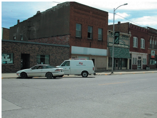
Existing east side of downtown.
